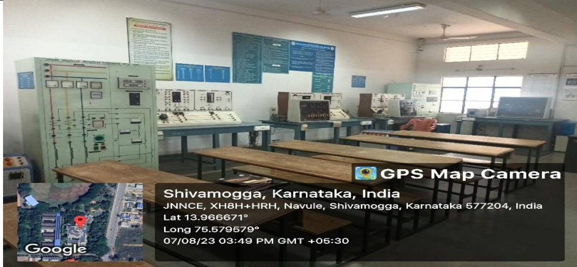
Pic 6:Basic Electrical Engg Lab
